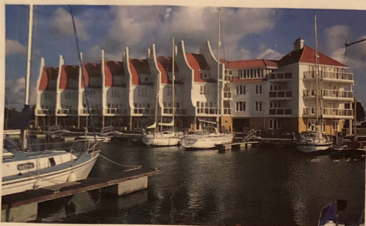
Above: Moriconium Quay – marina development, Hamworthy
