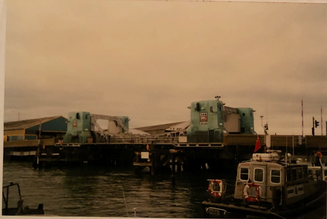
Poole's third bridge, built in 1927 at a cost of £50,000 and lifted by electric
